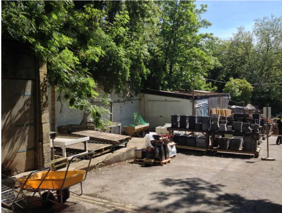
Existing brick structures used for storage
